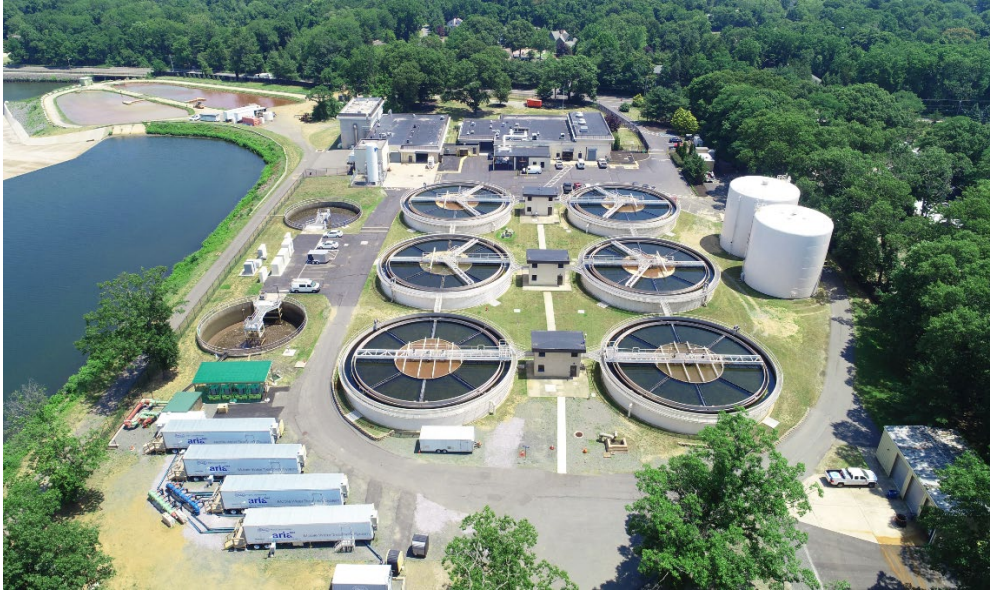
Pictured: New Jersey American Water's Swimming River Water Treatment Plant in Colt's Neck, NJ
