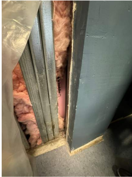
Photo 3 : Probe 1, interior of wall opposite of probe. Completed by others.
